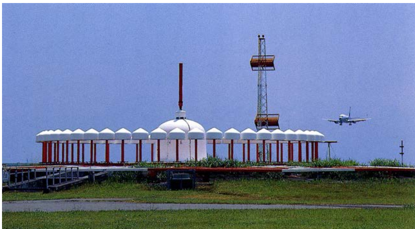
Photo 2 Doppler VHF omnidirectional radio range beacons and distance measuring equipment
