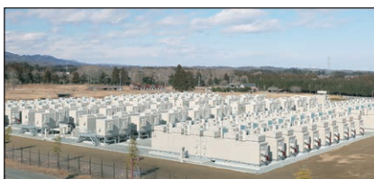
Tohoku Electric Power Co. Inc. Battery System for Substation
