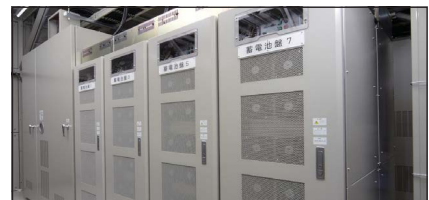
TOBU Railway Co. Ltd. Regenerative Battery Device
