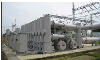
500kV Gas Insulated Switchgear
