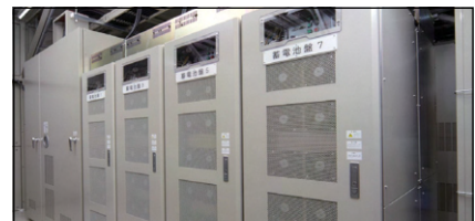
TOBU Railway Co. Ltd. Regenerative Battery Device
