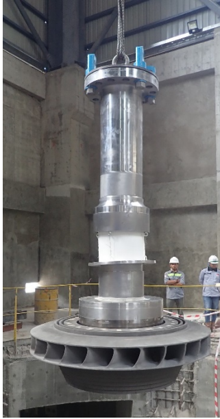
(Photo) Similar Francis turbine as for the Kerinci Hydropower Plant
